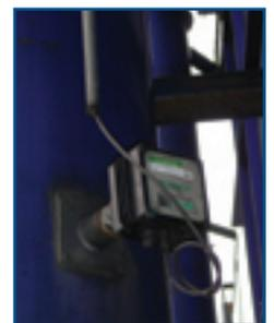
Electrodynamic Sensor installed in bag house outlet
