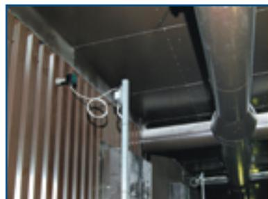
Electrodynamic sensor installed directly in Baghouse compartment wall
