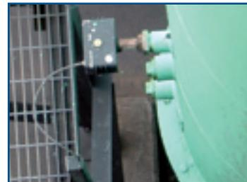
Pro-Scatter and Electrodynamic Main Stack Sensors
